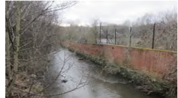
3. View of River Medlock looking South
