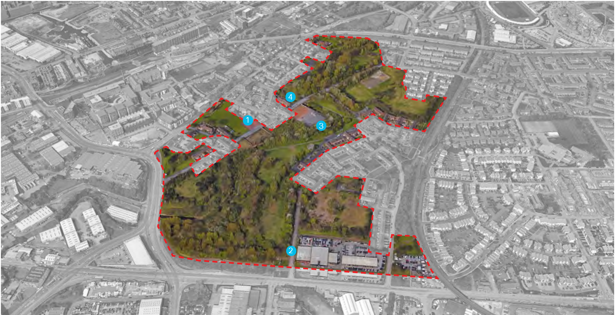
Figure 7.9 Aerial view of the regeneration area from south
