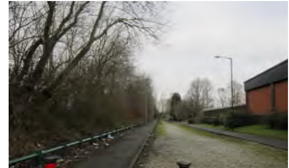
2. View North along Limebank Street
