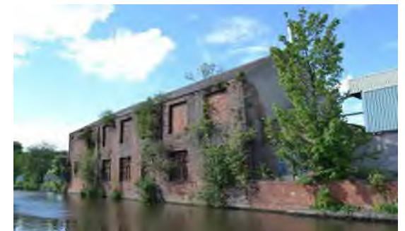
4. View of canal side warehouse
