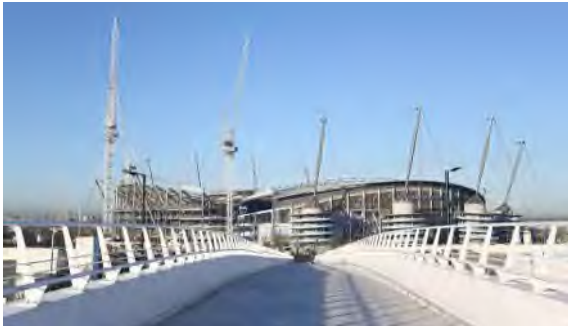
2. View of Etihad Stadium from the CFA bridge link
