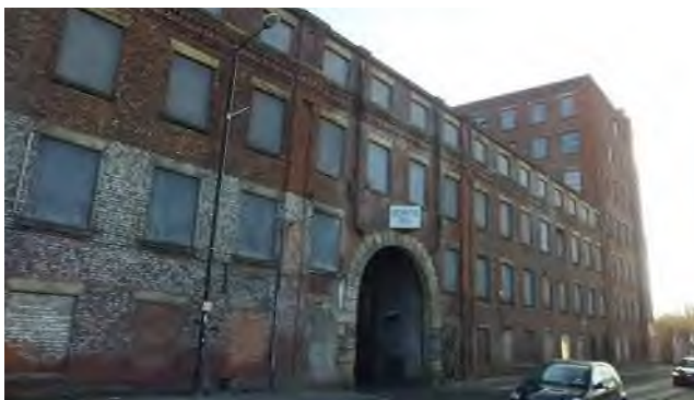
2. View of Brunswick Mill frontage onto Bradford Road
