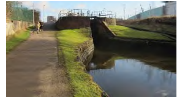
2. View of canal lock looking East
